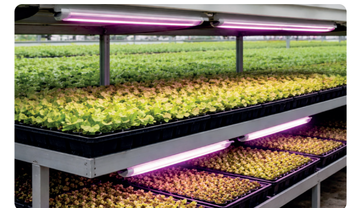
Figure 2 | underbench setup with +/- 90 cm height between crop and lights.
